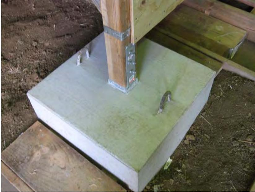
**Figure 19: Typical Retrofit 2 Footing**
