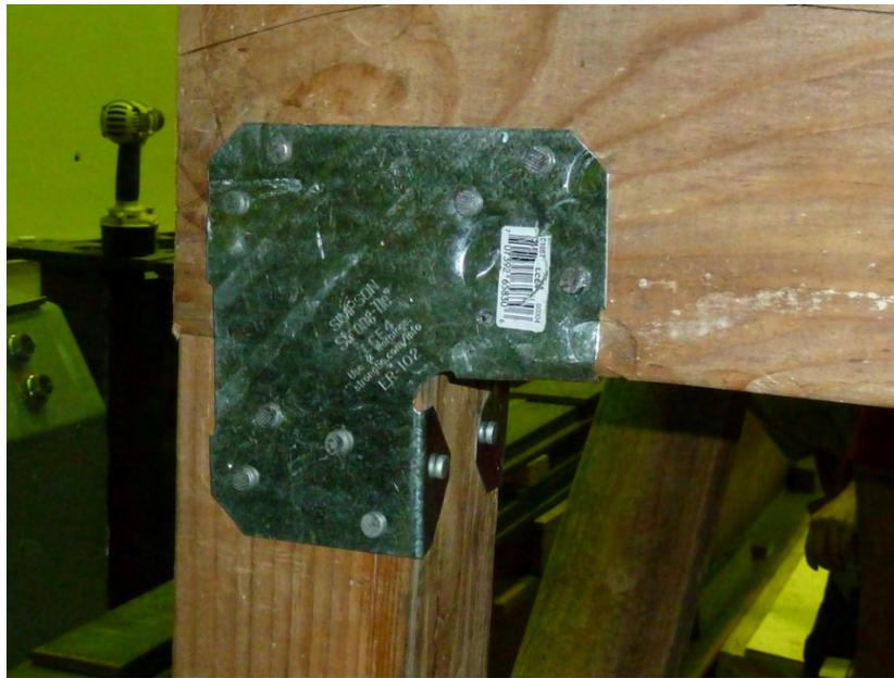
Figure 16: LCE4 Post Cap Installed on 4x4 Post
