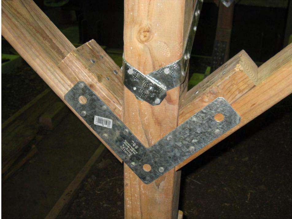
Figure 11: Typical Retrofit Scheme 1 center post with Simpson 88L strap installed
