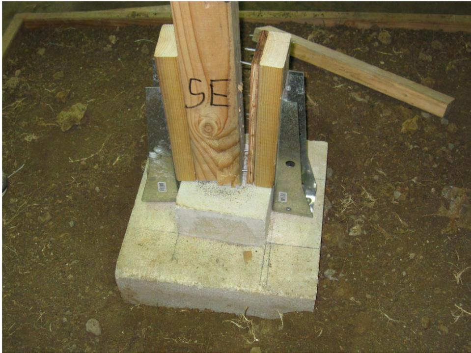
**Figure 45: HDU5 separation from 2x4 Blocking Separation From 4x4 Posts**
