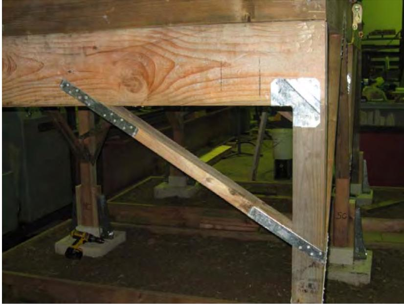
**Figure 13: Typical Retrofit 1 corner post with HRS12 straps installed**
