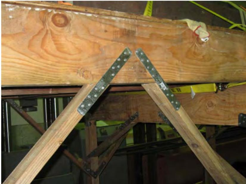
**Figure 14: Typical 2x4 diagonal brace retrofit with HRS12 straps installed**
