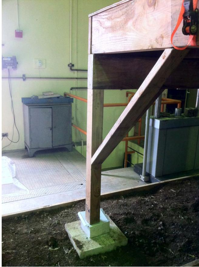
Figure 3: Typical 2x4 Diagonal Brace with toe-nail connections
