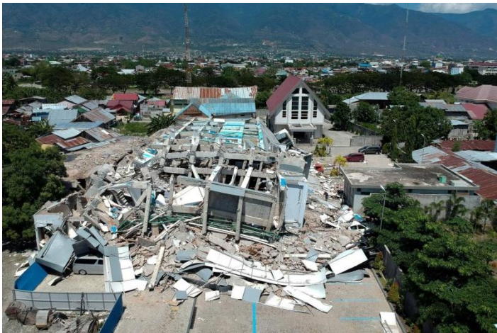
Collapse of 7 story Roa Roa Hotel due to earthquake shaking
